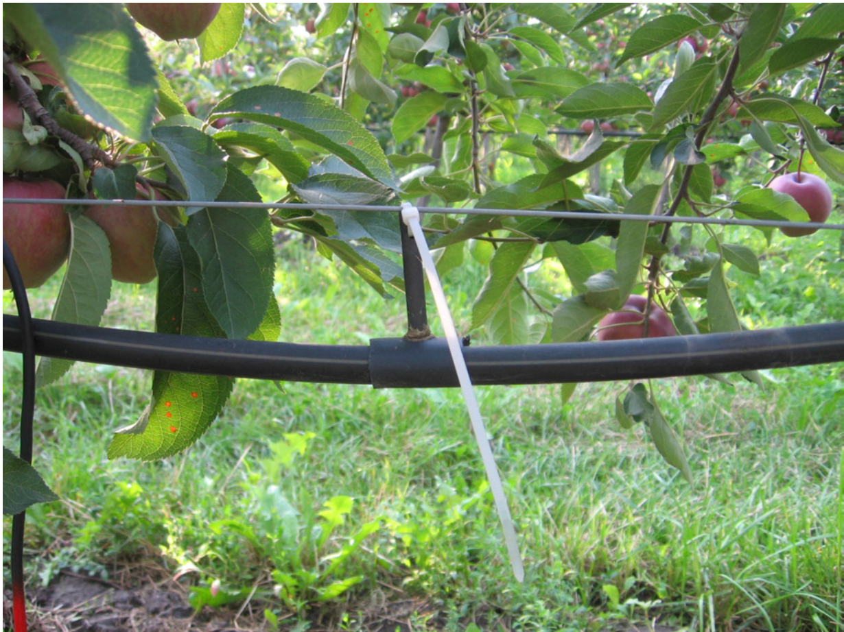
Figure 7. Detail of the drip hose bending over the location of the soil moisture sensors
